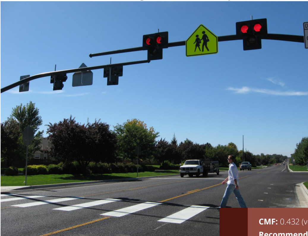
Figure 21 Pedestrian Hybrid Beacon
