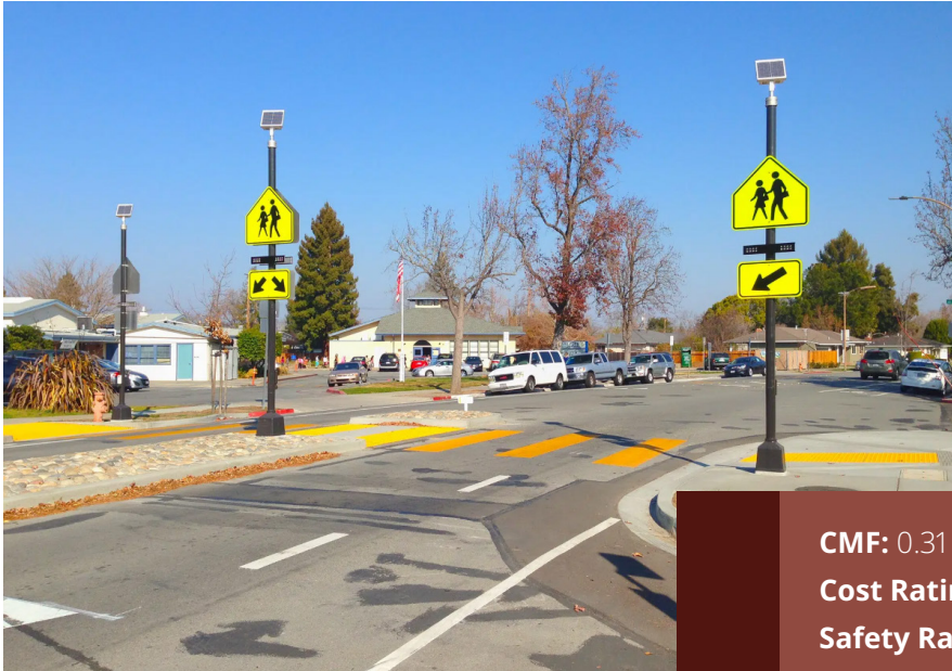
Figure 29 Rectangular Rapid Flashing Beacons
